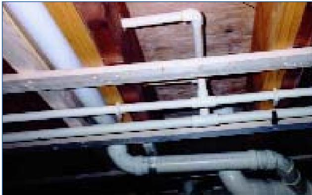
said Barucci. "Whenever I bid for spec work, I show the alternative and compare the job costs using copper vs. CPVC. If we're doing design/build business, we automatically specify FlowGuard Gold CPVC pipe and fittings. It's so much easier. There's no cleaning or soldering. You just snip and glue. The speed is incredible."
