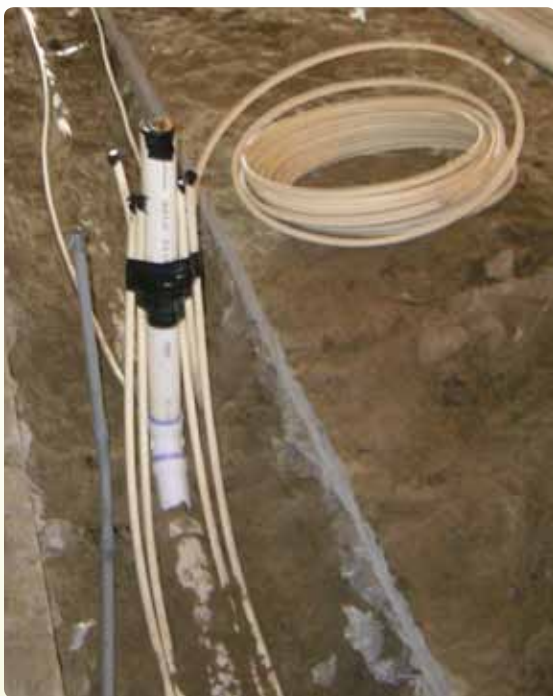
FlowGuard® Bendable composite pipe is easily installed in new construction from a large coil.
