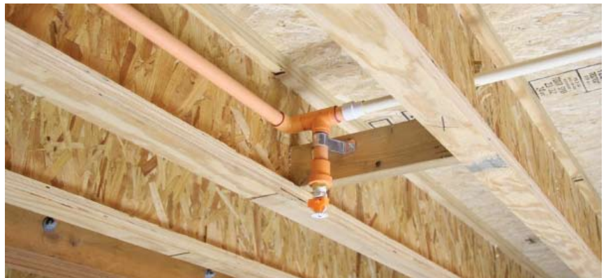
A BlazeMaster multipurpose residential fire sprinkler system. (Photo courtesy of The Lubrizol Corp.)
