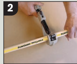
Cut the FlowGuard® Bendable pipe using a standard pipe wheel cutter
