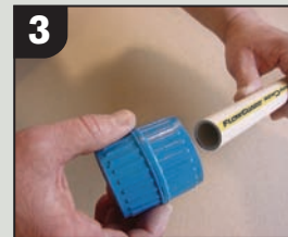
Deburr the FlowGuard Bendable pipe
