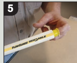
Install the sleeve fitting into the FlowGuard Bendable pipe and twist it slightly
