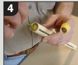
Cement the outside diameter of sleeve fitting and the inside diameter of the FlowGuard Bendable pipe
