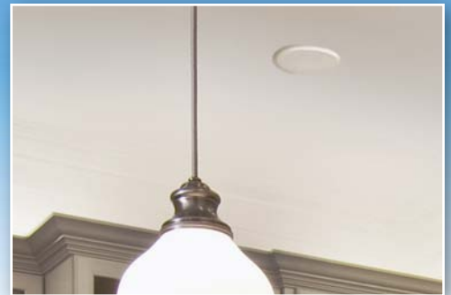
Modern installation with concealed sprinkler heads.
